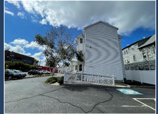
Handicap Accessible Ramp
